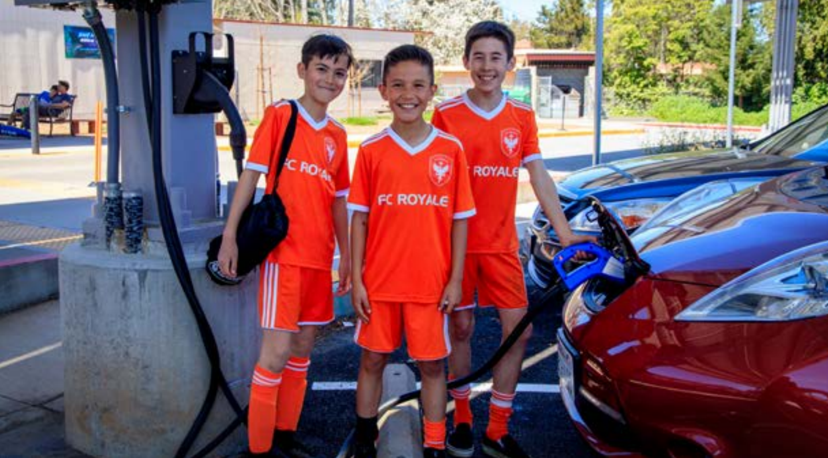
Solar canopy at elementary school powers classrooms and provides electric vehicle charging capacity Photo Credit: Frank Spada
